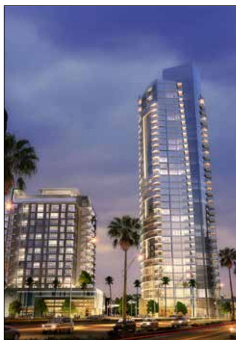
Once complete, the Shoreline Gateway Tower will be the largest building in the city of Long Beach.
