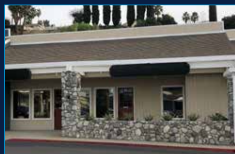
Left: The exterior of the new District 6 Union Hall in the San Gabriel Valley. The facility is still under construction and is expected to open in mid May at 830 N. Diamond Bar Blvd., Diamond Bar, CA 91765.
