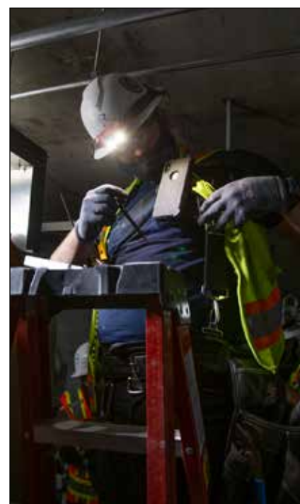
More than 30 Local 11 electricians are working on the job.
